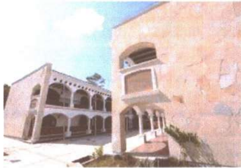
F3: Fachada principal
