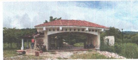
F3: Fachada principal
